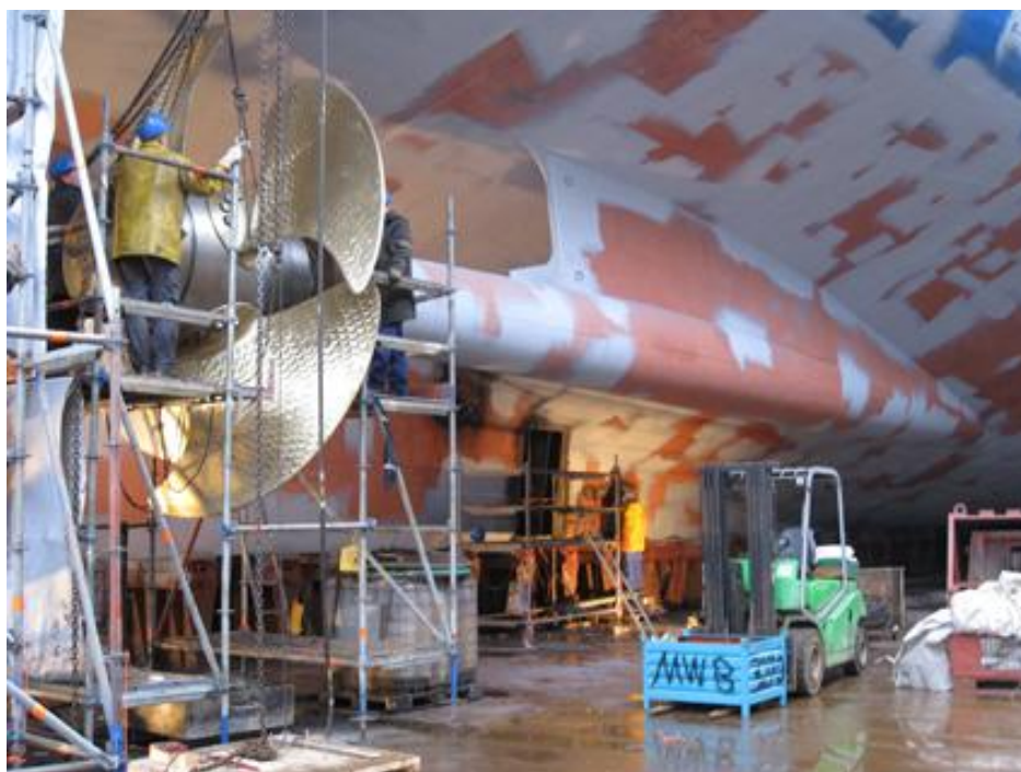
PrimeServ engineers fitting the M/V Sassnitz's new propeller blades
